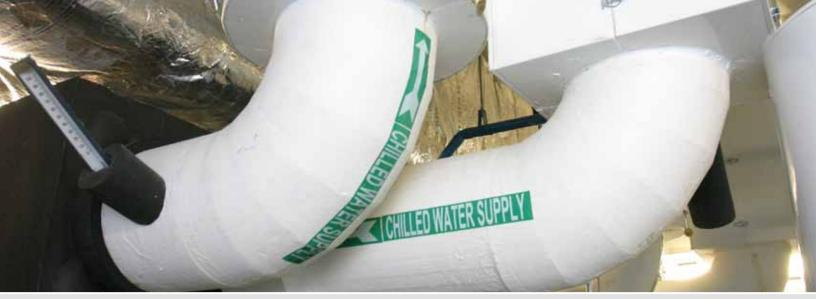
Chilled water distribution lines protected with FOAMGLAS® insulation can withstand high humidity and physical abuse.
